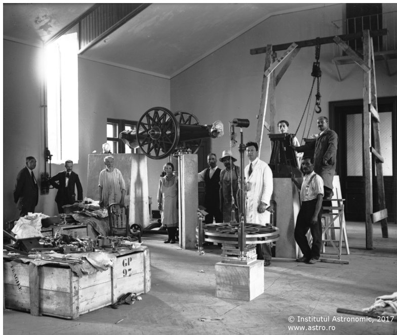
Fig. 1 – Team of scientists and workers during the installing of the Gautier-Prin telescope in the Meridian Hall of Bucharest Observatory (1926).
